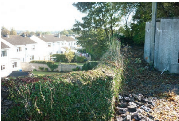
Fig. 21 View of wall head to castle bawn retaining wall.
