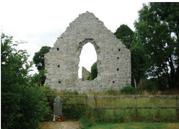
Fig. 33 View of recent conservation repairs to east gable of Grey Abbey.
