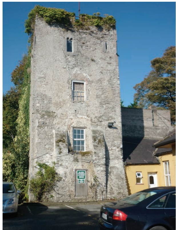
Fig. 22 View of the east side of the Gatehouse.
