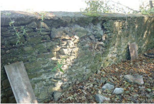
Fig. 63 View of damage to castle bawn wall showing fallen masonry.
