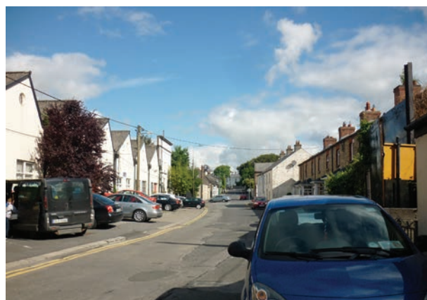
Fig. 25 View looking north along Cleamore Road.
