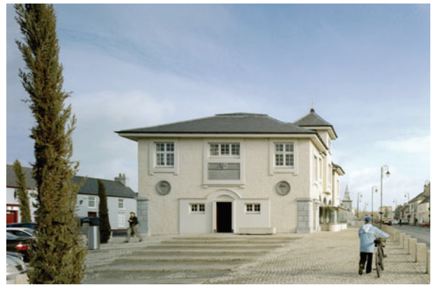
Fig. 74 View of hard landscaping and conserved market house at Abbeyleix, Co. Laois.
