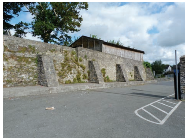
Fig. 69 View of car park along the base of the cathedral enclosure wall.
