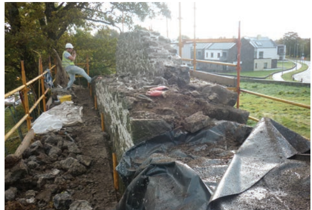
Fig. 48 View of conservation works being undertaken at Atherny, 2014.
