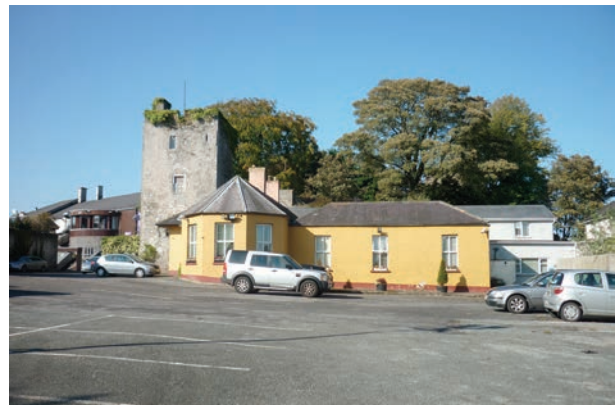
Fig. 46 View across car park towards Leinster Lodge and Gatehouse.
