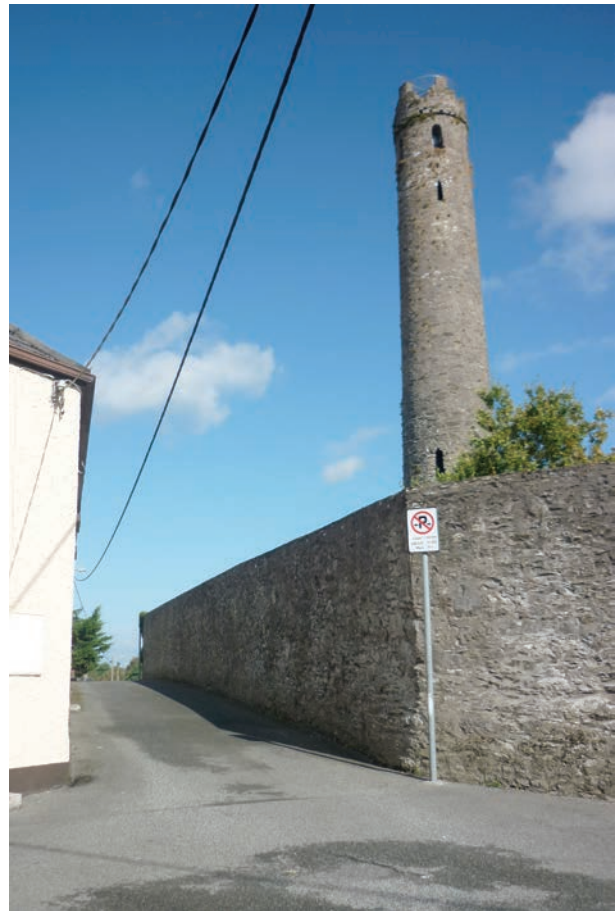
Fig. 18 View of outer face of cathedral wall at Firecastle Lane.
