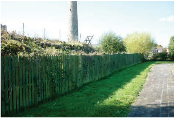
Fig. 64 View of palisade fencing in gap to cathedral wall, with fallen masonry visible in undergrowth along sloping bank.
