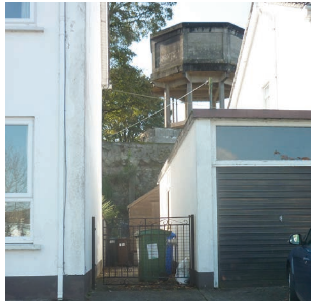
Fig. 44 View from Dara Park towards castle bawn retaining wall.
