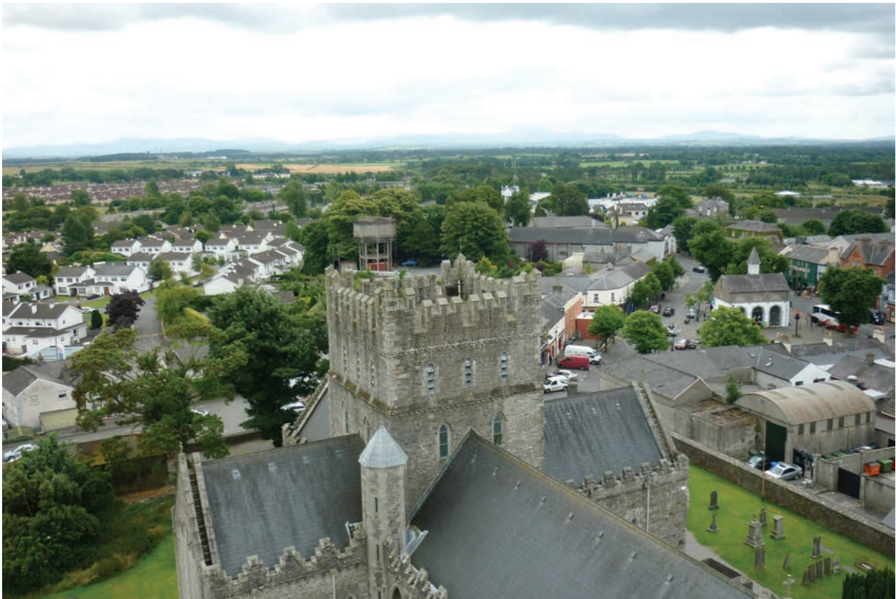
Fig. 38 View over cathedral towards castle site and water tower, taken from round tower prospect.
