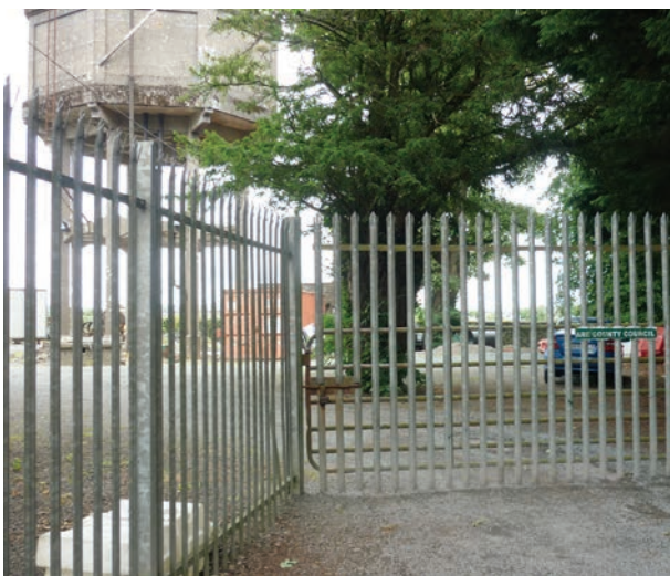
Fig. 43 View of gates to entrance to council yard at Castle site.
