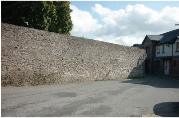
Fig. 27 View along cathedral enclosure wall on Chapel Hill.
