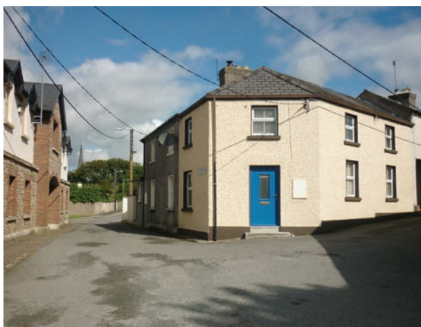
Fig. 23 View looking west along Fire Castle Lane.
